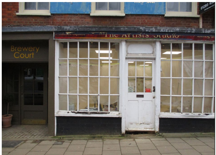
The shopfront, and entrance to Brewery Court
