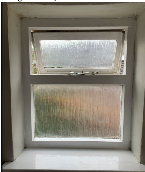
First floor window (to toilet)
