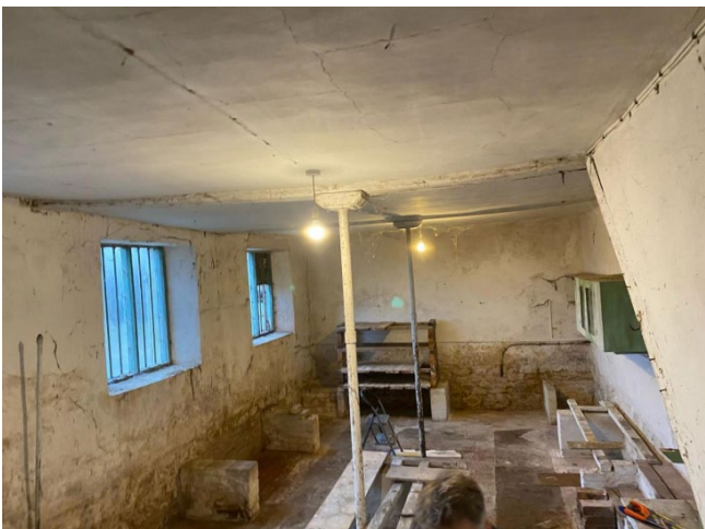
The former dairy with ceiling props
