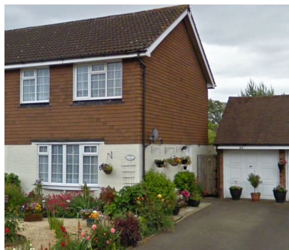
House front and south side, and garage
