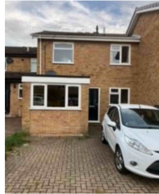
Existing view of front elevation
