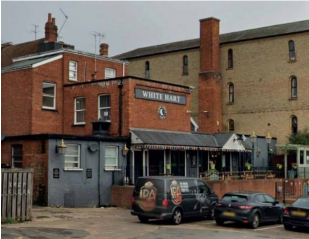
Existing signage – rear elevation
