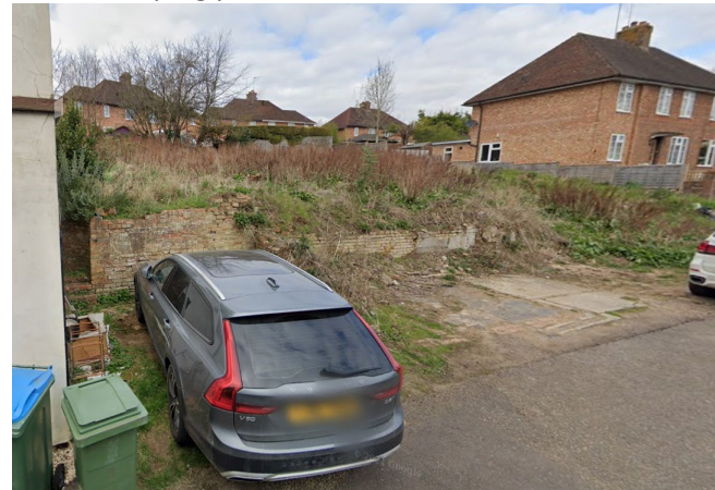
The site from the south showing remains of buildings and access to rear of Bath Lane cottages (between rendered cottage and retaining wall and car)
