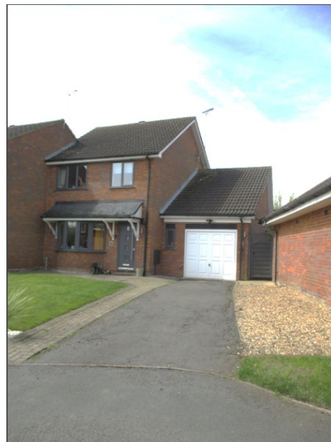
The front elevation (13/4/24). The building on the right is the garage block for the five houses.
