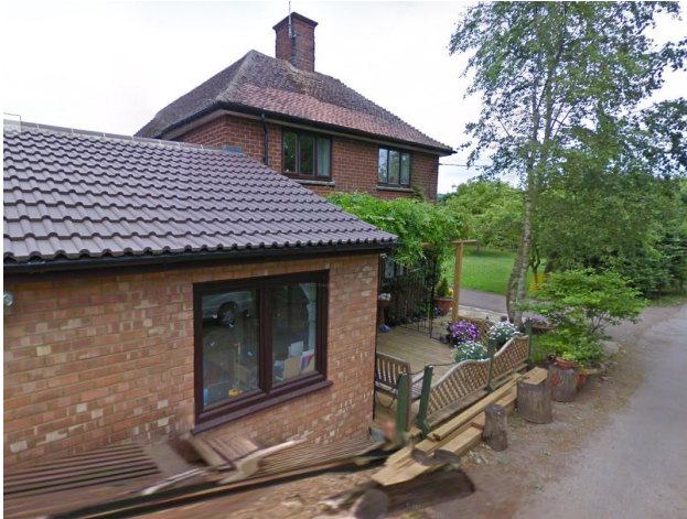
Part of the extension, the house, and the lawned area (these 3 photos Google Streetview 2011)
