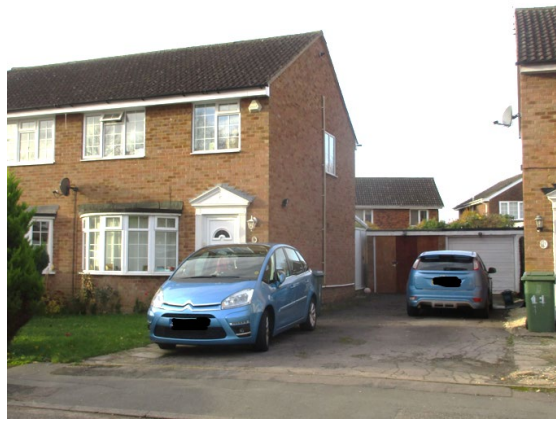
House front and garage (taken 24/11/23 for previous application)
