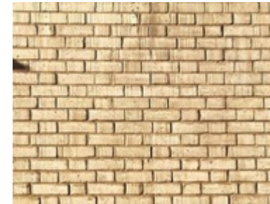
Yellow bricks laid in Flemish bond
