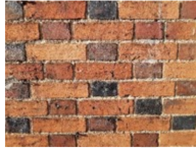
Flemish bond with vitreous headers
