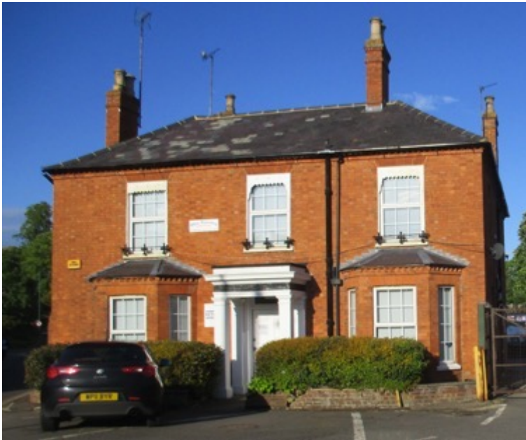
Wharf house western elevation
