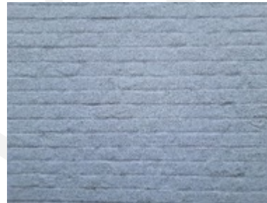
Painted English bond brickwork
