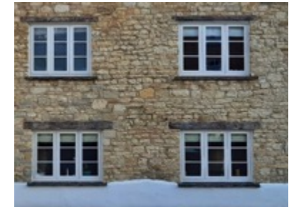
Coursed limestone rubble
