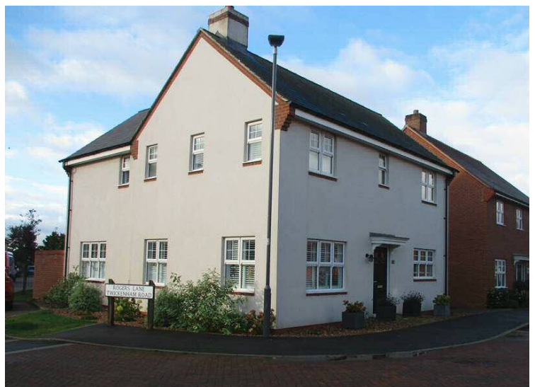
General view of house front and side
