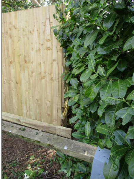
Land behind fence, formerly 'lawn'
