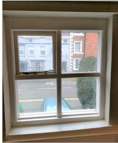
Existing window interior (from D&A Statement)
