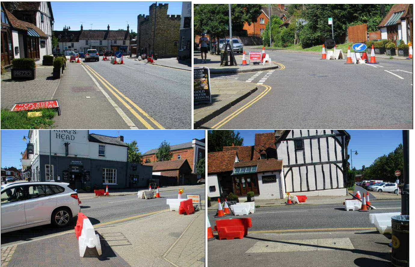
The crossing as existing (7/8/20):
