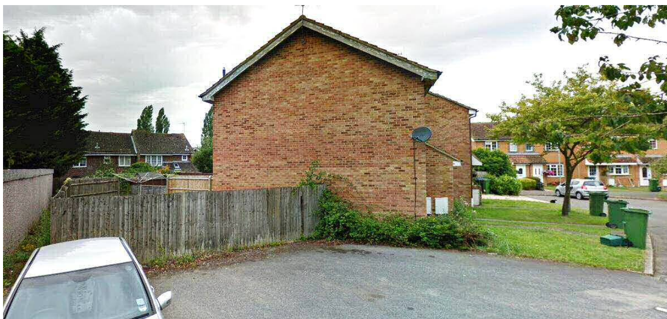
Side view showing garden fence and shared pathway to left between fence and Bodenham Close garages, and public parking area.
